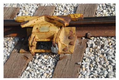
**40.2** Derails must be installed when there is any possibility of equipment that has been left standing on tracks other than main tracks or sidings being moved by gravity so as to obstruct a main track or siding.
